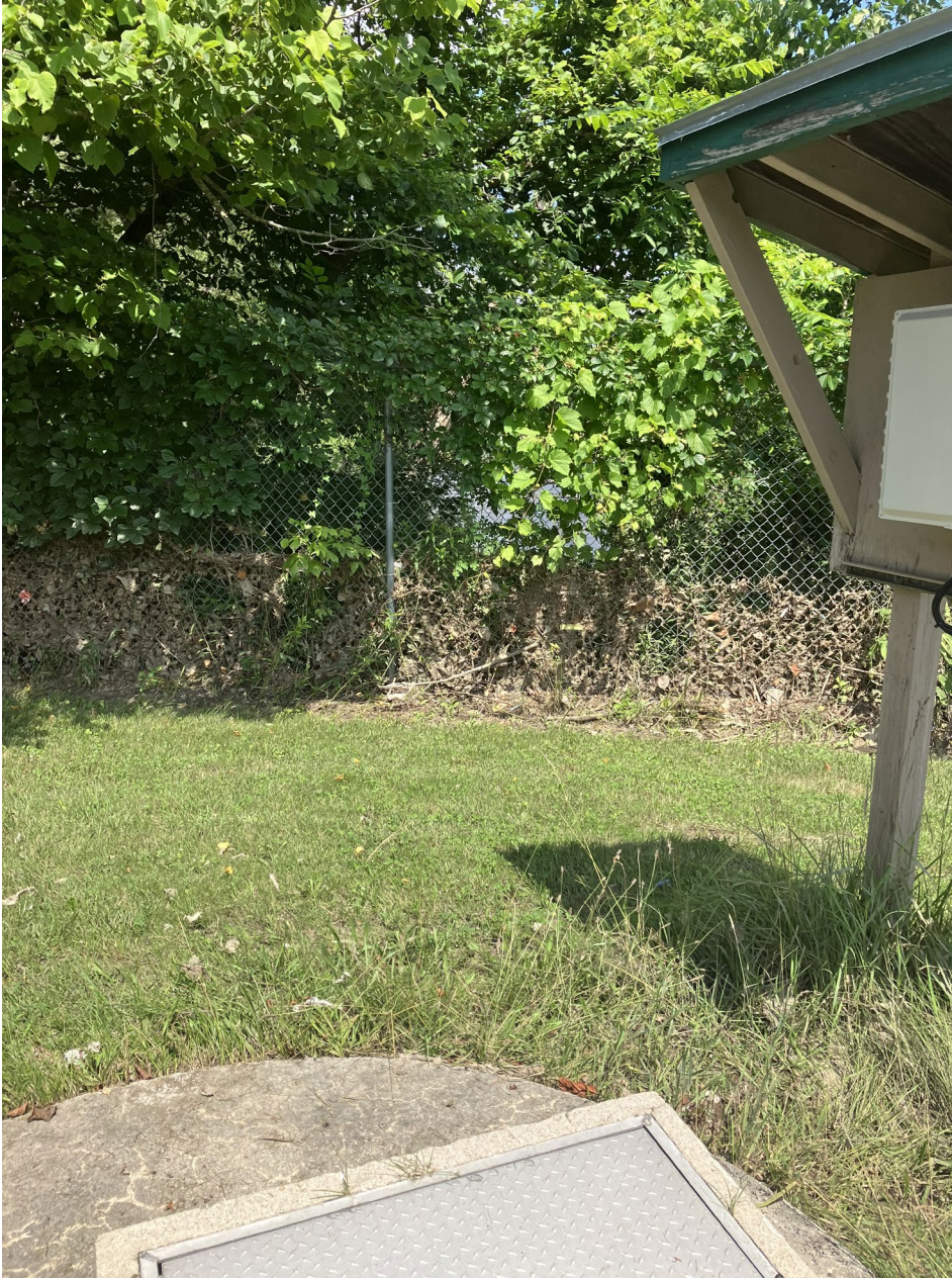
1- Perimeter Fence Showing Debris From High Water and Influent Pump Station
