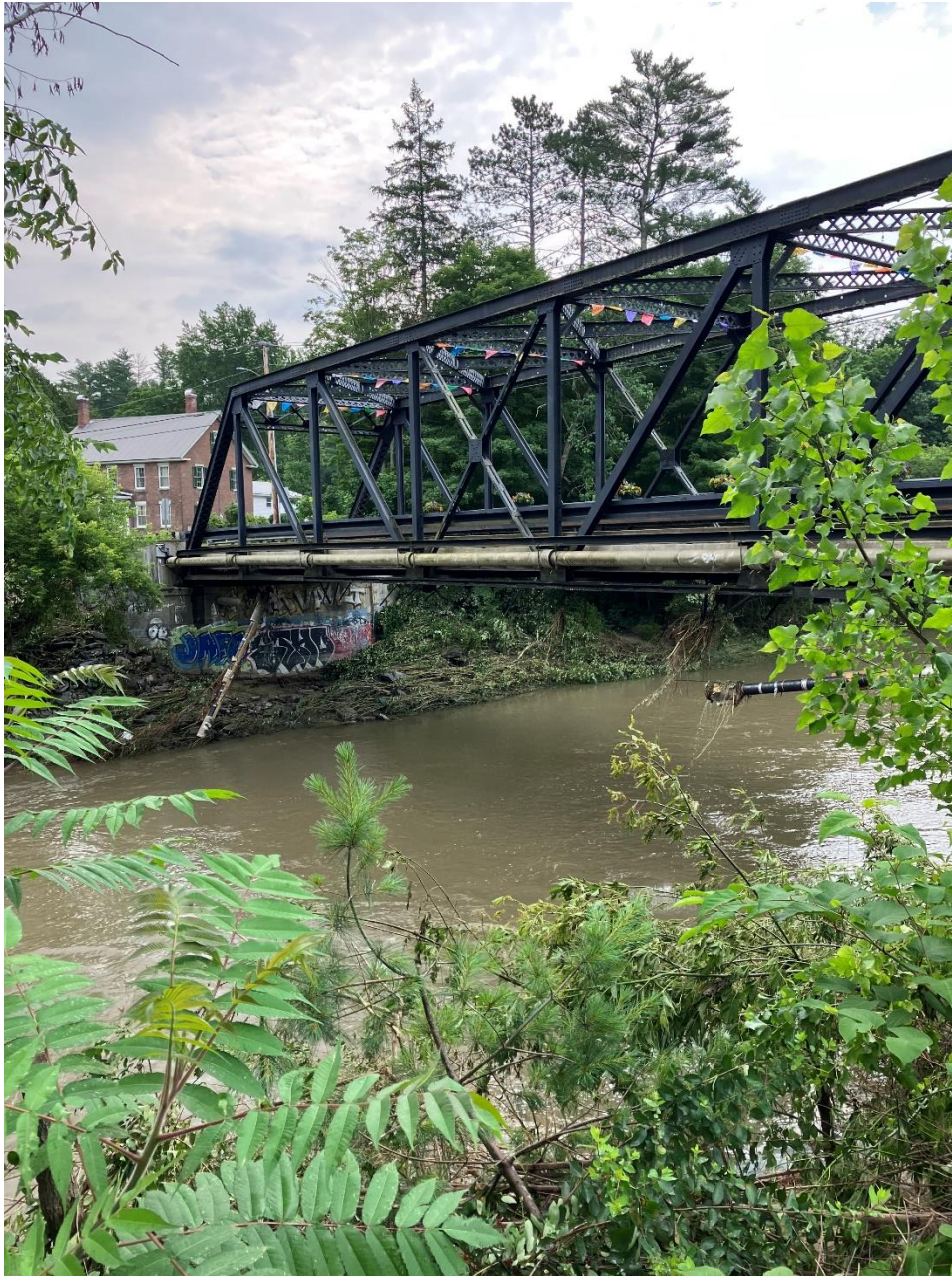
29- Railroad Street Bridge Severed 8" DI Sewer Crossing
