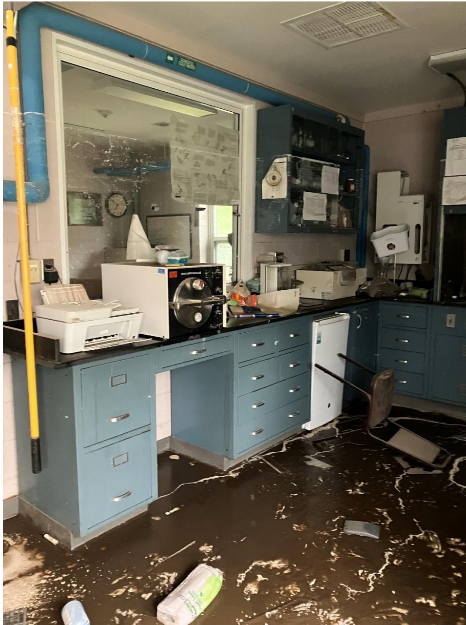
2- High Water Mark in Laboratory Area
