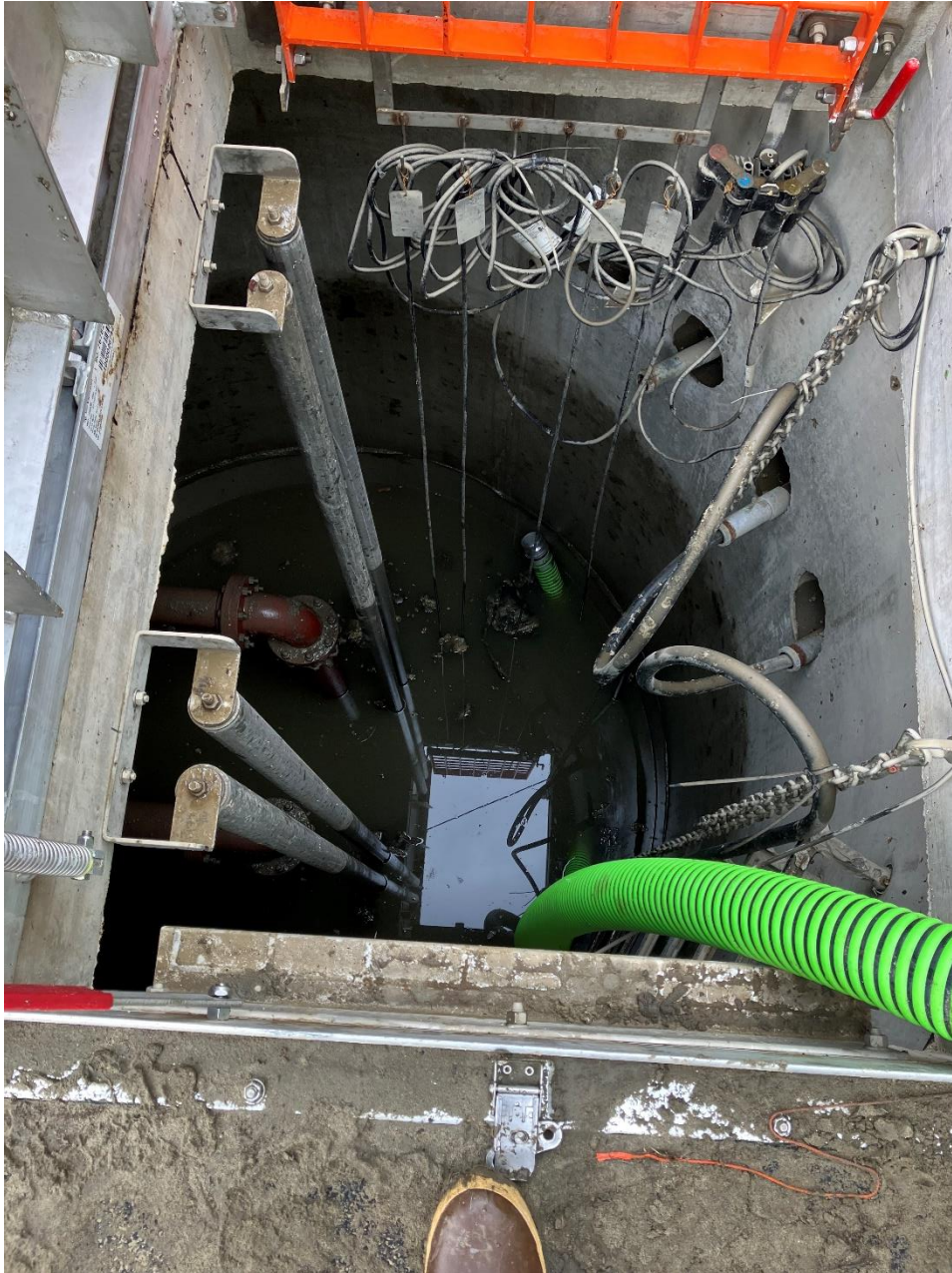
25- Interior View of River Road West Pump Station Wet Well
