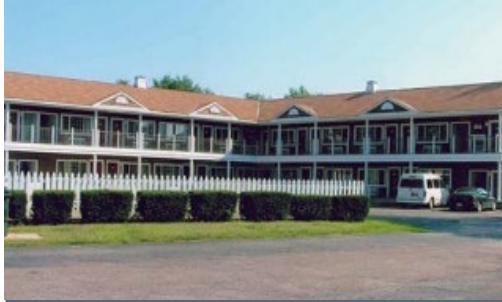
Braeburn Apartments South Burlington
