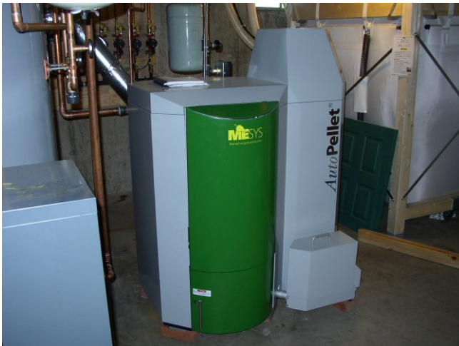
Figure 10: SSREIP supported Pellet Boiler installed at Burke Mountain Academy. Photo by Cutting Edge Energy Systems
