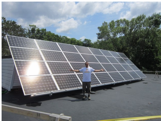
Figure 6: 8.9kW PV system installed on the Wallingford Elementary school
