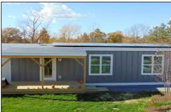
Figure 1: Net Zero home (with PV system supported by the SSREIP)
