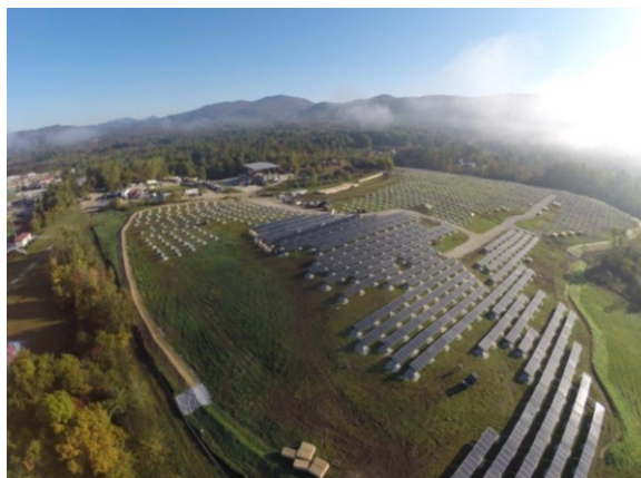
CEDF provided grant funds to support the Stafford Hill Solar Energy Storage Project in Rutland.
