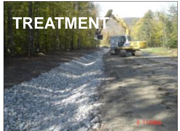
Ditch stabilization saves road and reduces erosion
