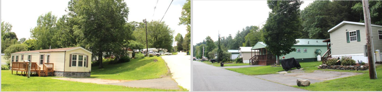
Figure 18. Angled units in the upland portion of the park (left) and perpendicular to the road in closer arrangements in the flat portion of the park (right).
