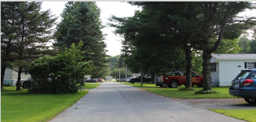
Figure 49. View of the Tucker Mobile Home Park including streetlights, driveways, and landscaping.
