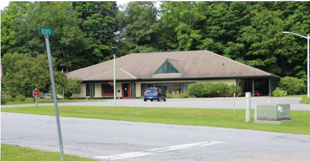
Figure 43. The community center at Williston Woods.
