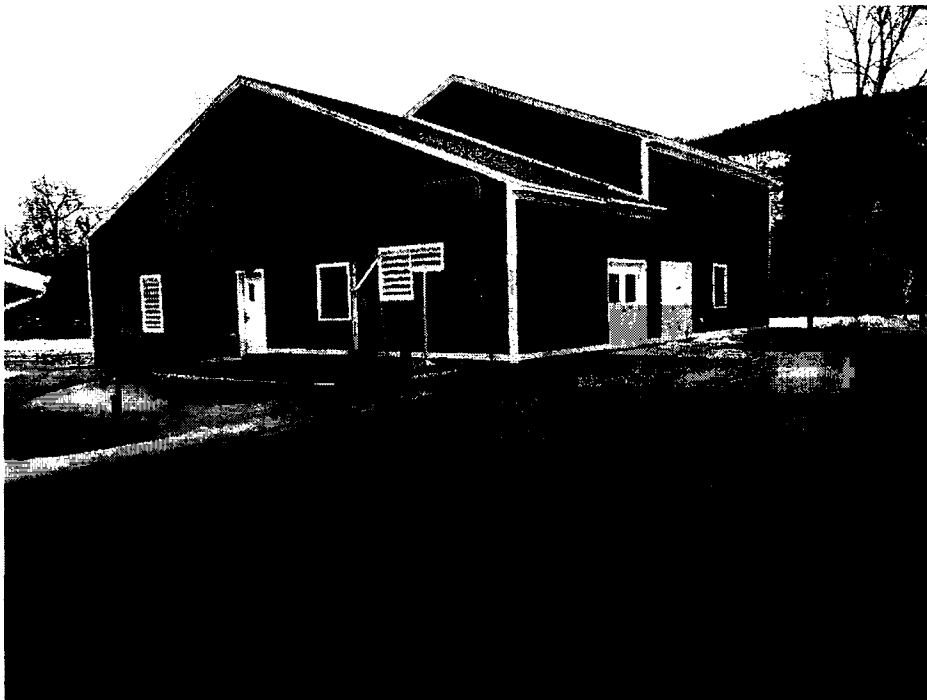
Figure 2: New process building housing CoMag® system for improved phosphorus removal.
