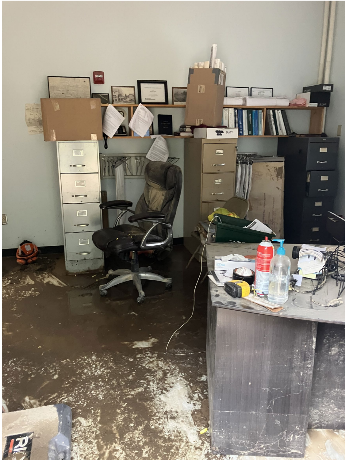
28- Main Control Building Office.
