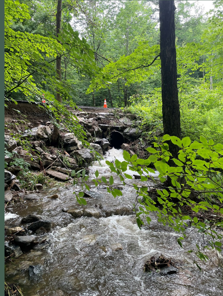
North Branch Rd- significant shoulder issues and undersized culverts
