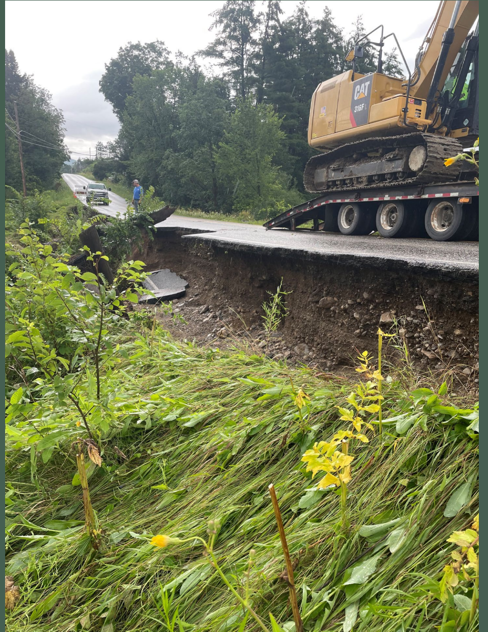
Figures 1 & 2: Shoulder/ Road Failure- Painter Rd.
