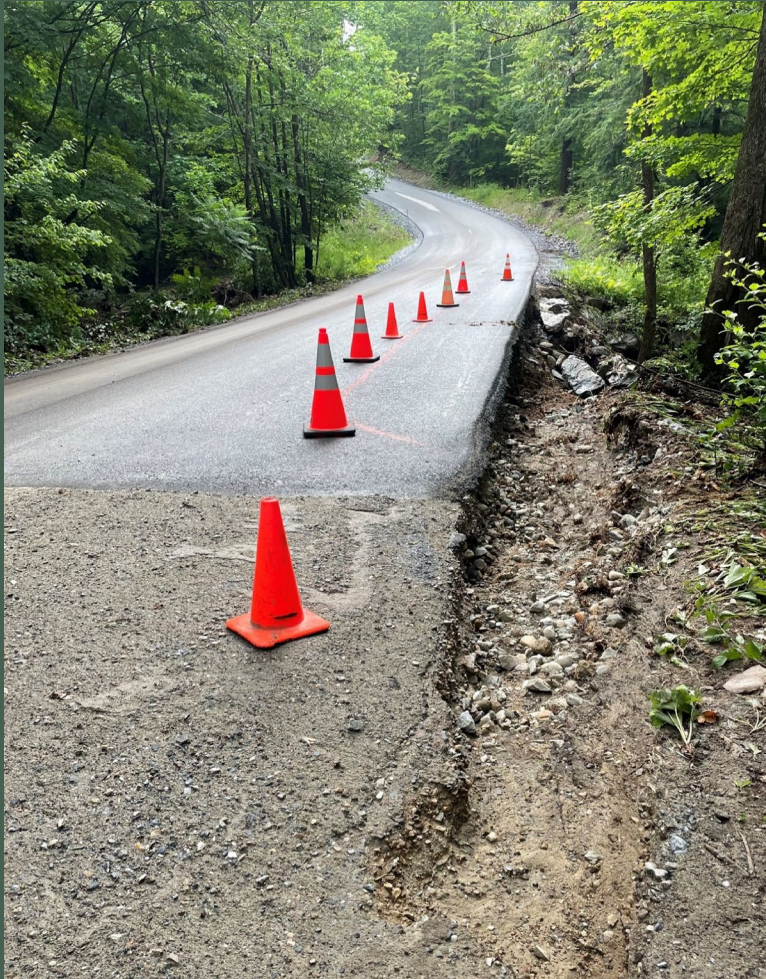
North Branch Rd- significant shoulder issues and undersized culverts
