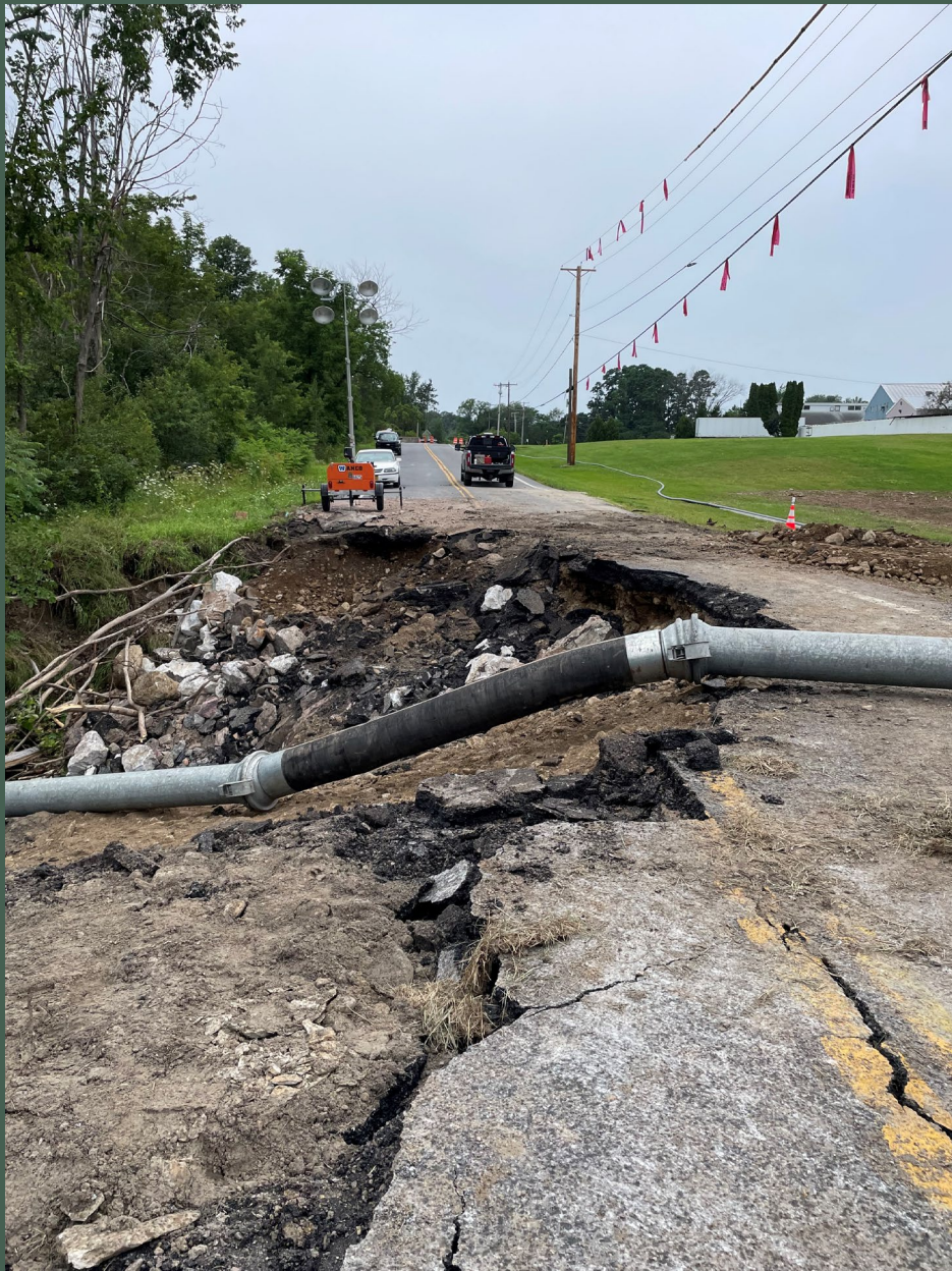
Figures 1& 2: Dow Pond- Water Line Break and Rt. 116 Failure
