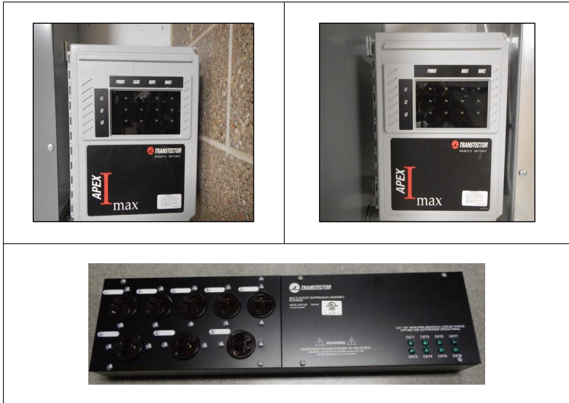
Figure 3e Surge Protection Device
