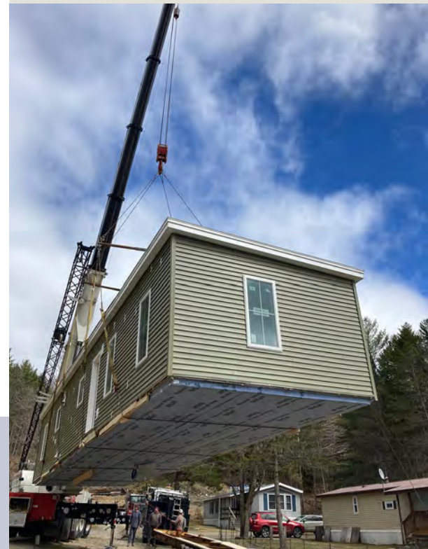
A zero-energy modular home being placed at Evergreen Mobile Home Park in Hardwick by the Lamoille Housing Partnership.
