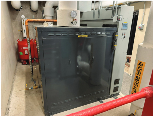
Electric boiler
