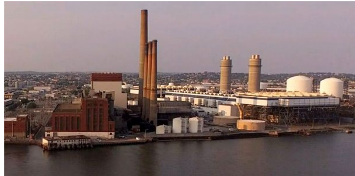
Mystic Generating Station in Everett, MA
