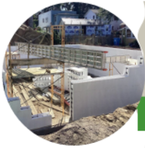
Home under construction in Burlington's Old North End
