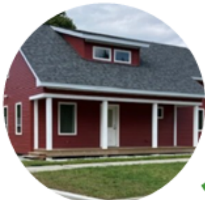
First home completed in Rutland
