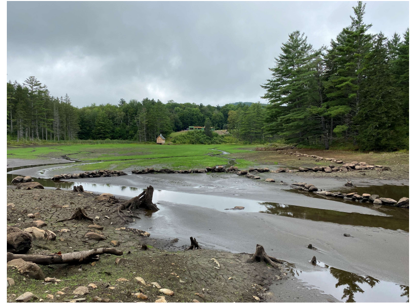
Lyons Pond Dam, Peru, LOW Hazard
