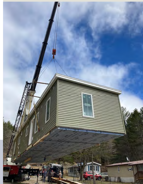
A zero-energy modular home being placed at Evergreen Mobile Home Park in Hardwick by the Lamoille Housing Partnership.
