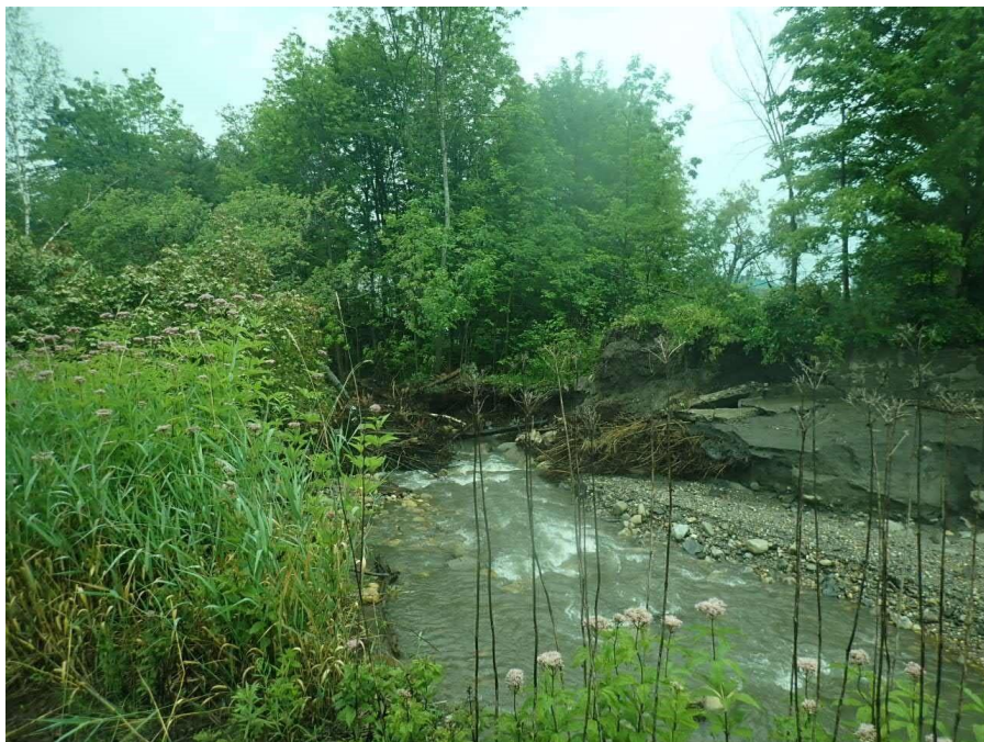
Hands Mill Dam, Washington, SIGN Hazard
