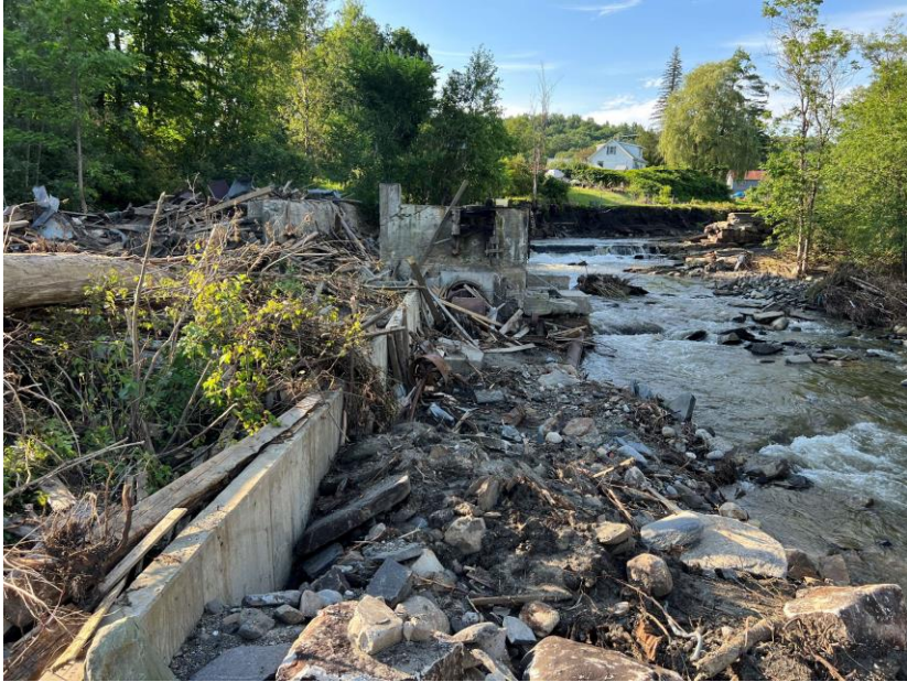
Clarks Sawmill Dam, Cabot, LOW Hazard
