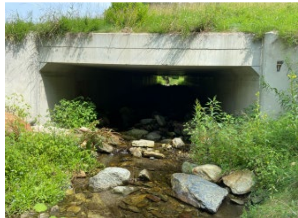
16' x 6' box culvert
