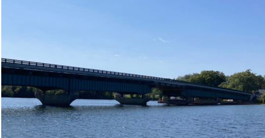
North Hero (Mother's Bridge) Bridge on US 2 After
