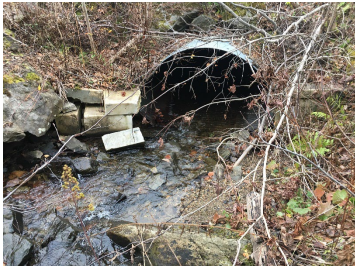
Killington Bridge 30 on US 4 Before
