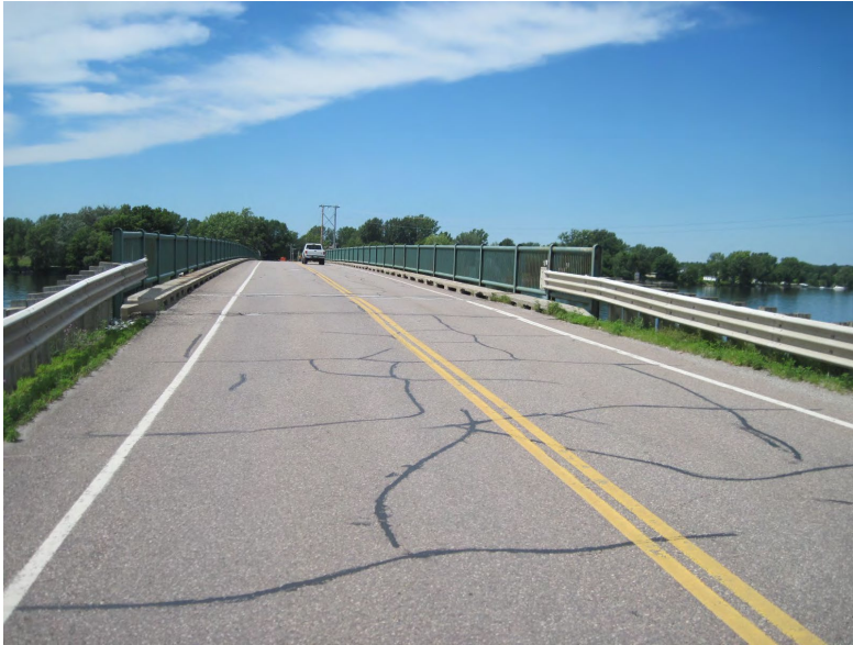
North Hero (Mother's Bridge) Bridge on US 2 Before
