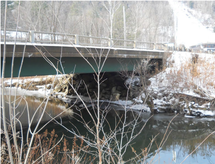
Killington Bridge 33 on US 4 Before
