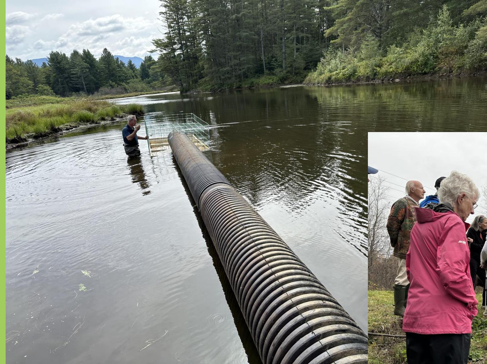
“Beaver Deceiver” installed in Cambridge Fall 2023
