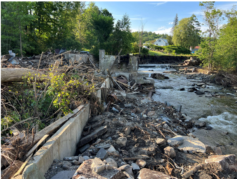
Clarks Sawmill Dam, Cabot, LOW Hazard
