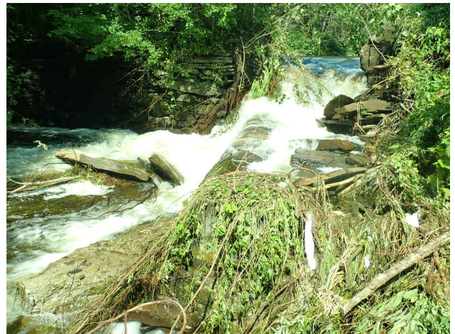
South Woodbury Pond Dam, Woodbury, SIGN Hazard
