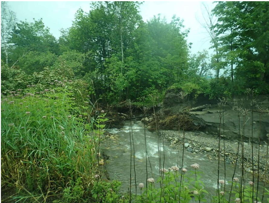
Hands Mill Dam, Washington, SIGN Hazard
