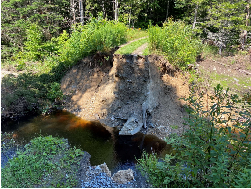
Quinn Lower Dam, Wallingford, LOW Hazard
