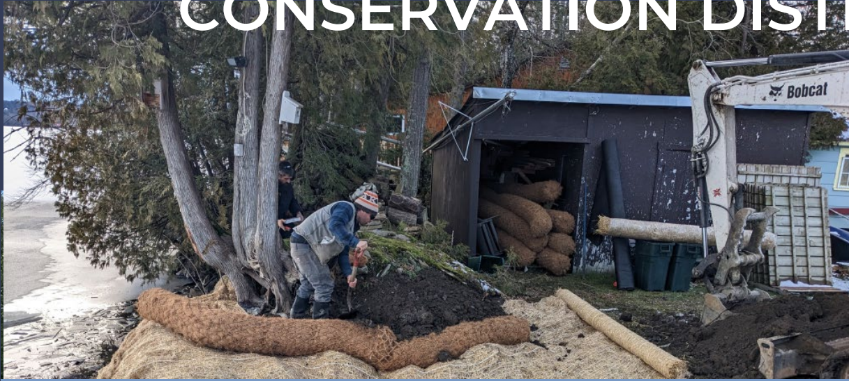
NATURAL RESOURCES CONSERVATION & RESTORATION
