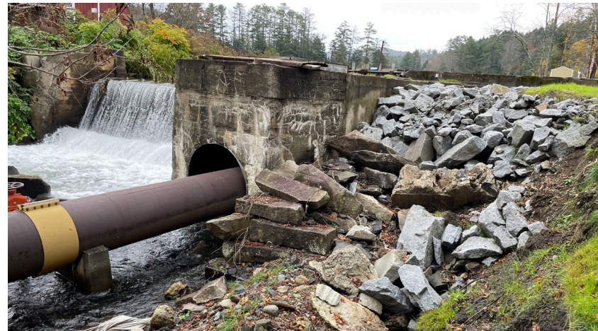
2023 Emergency Repair at East Calais Dam
