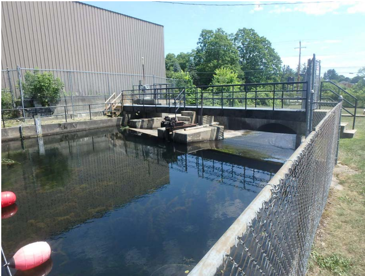
Lake Bomoseen Dam, Castleton
