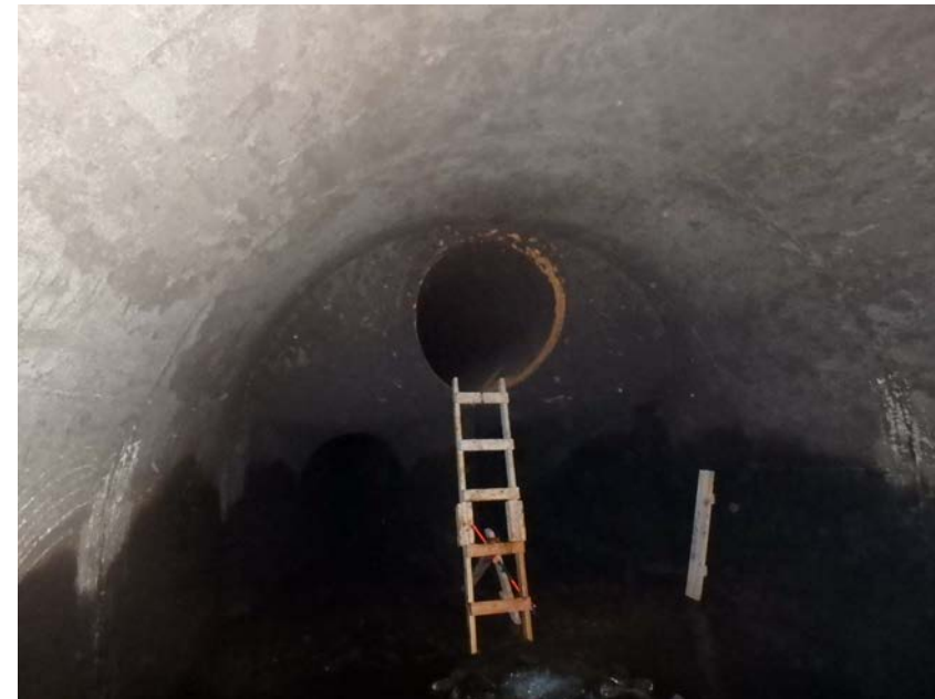
Waterbury Dam Tunnel
