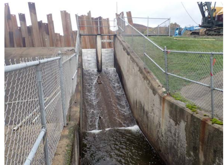
Miles Pond Dam, Concord
