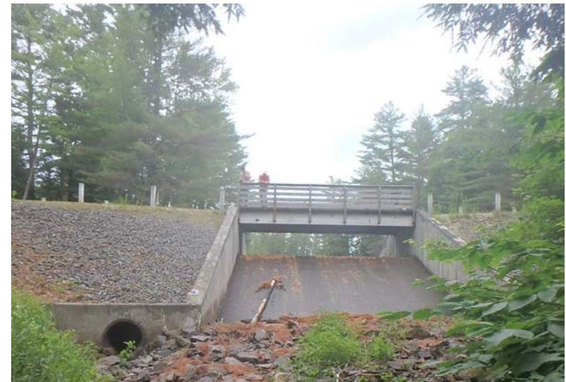
Lowell Lake Dam, Londonderry
