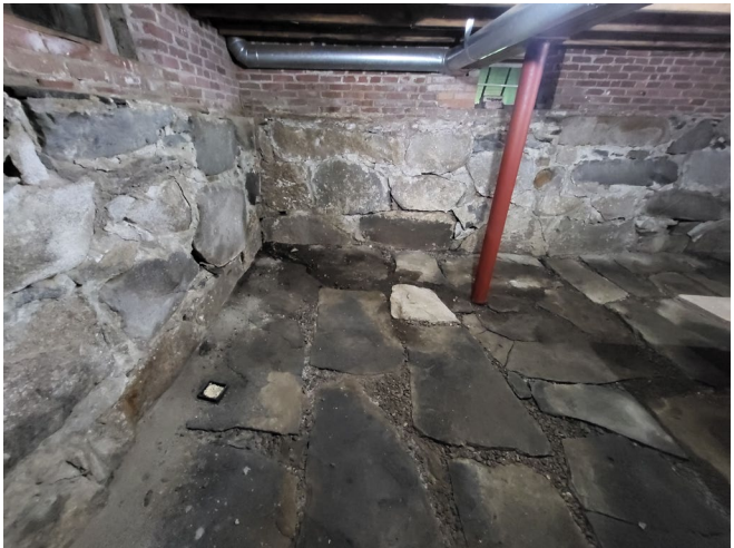
Morrill Homestead Basement
