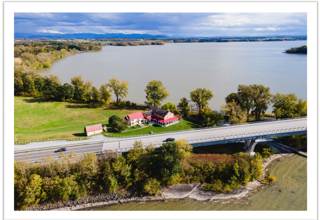
Chimney Point at Champlain Bridge, Addison 2023
