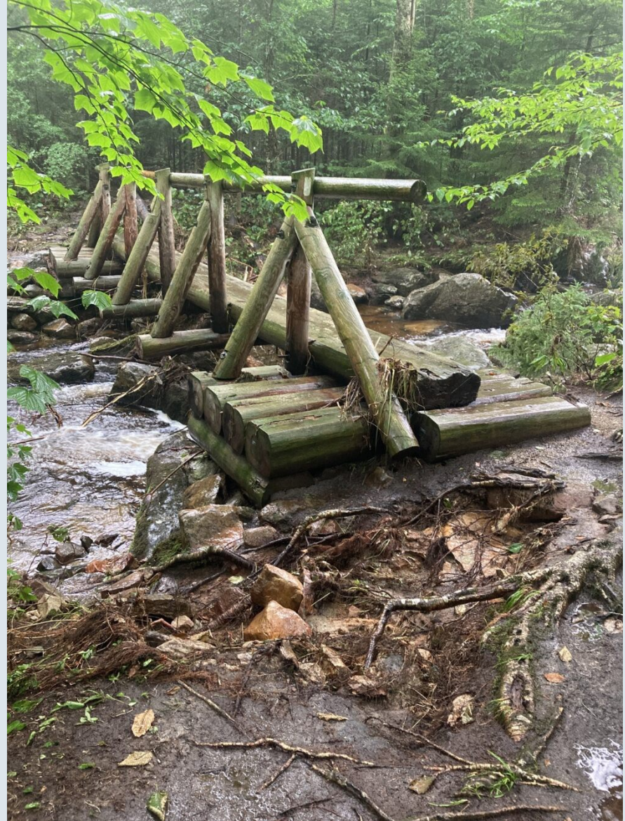
Gulf Stream Bridge - Woodstock
