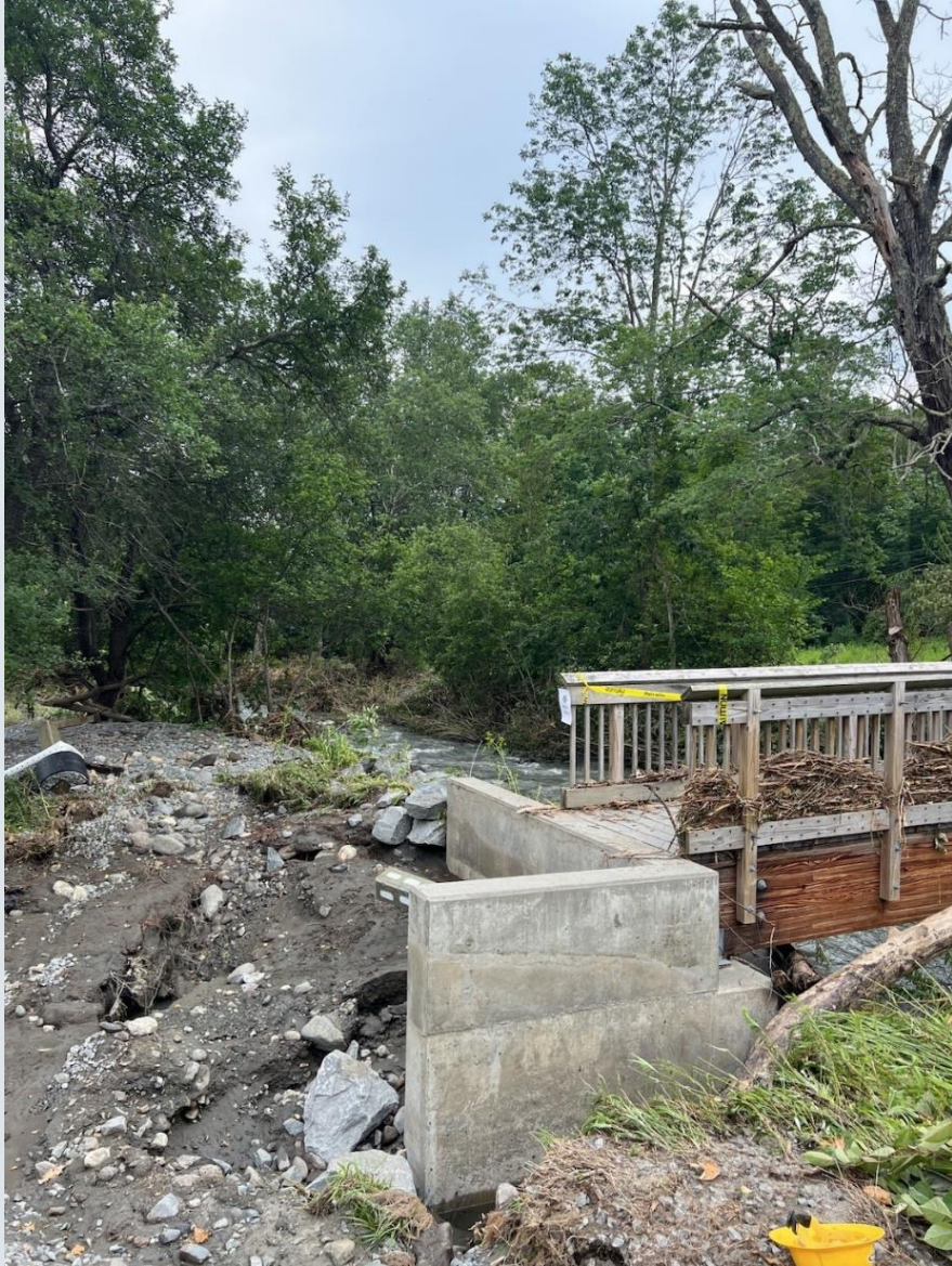
Homer Stone Brook Bridge - Wallingford
