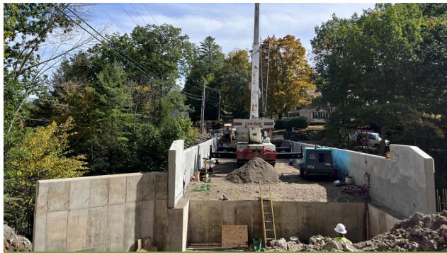
Construction and Maintenance
