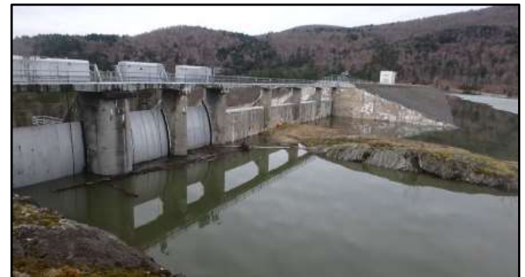
Waterbury Dam, Spring 2019 Flood Control
