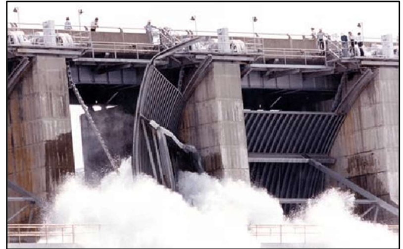
Folsom Dam Tainter Gate Failure, 1995
