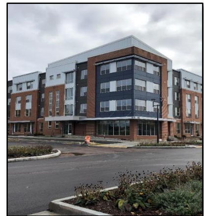
Garden Street apartments. Photo taken by VEPC staff.
