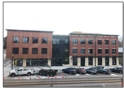
Completed redevelopment of Core Brownfield Site #3 – Congress and Main Streets. Photo provided by St. Albans City.
