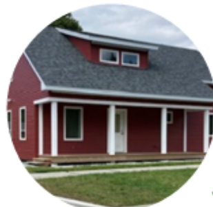
First home completed in Rutland
